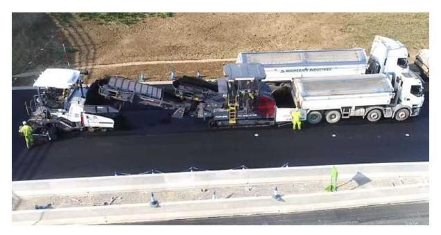
**Section 3:** The final layer of road surface is now being laid (see picture above) and white lines and other road marking will begin in the next few weeks. The last bridge over the A14 Huntingdon southern bypass, at New Barns Lane, is now structurally complete, with kerbing underway ahead of surfacing.
